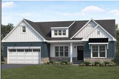
Upgraded Transitional B
